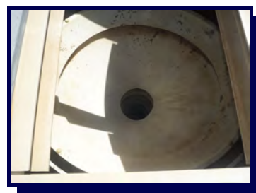
Grit Separator Unit (HeadCell)
