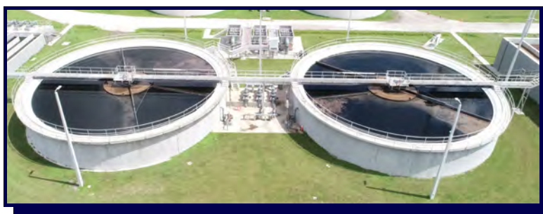
Secondary Clarifiers - IFAS BNR Treatment System
