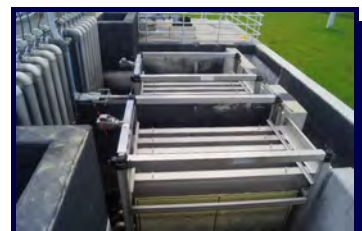
Tertiary (Disc) Filters
