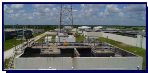
Carrousel BNR Treatment System: Anaerobic Basins
