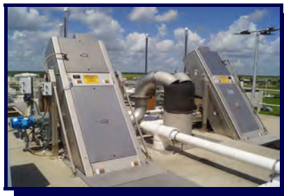
Mechanical Barscreens (3 mm)
