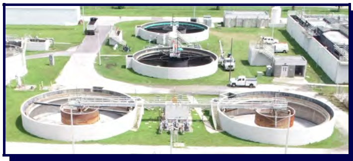
Carrousel BNR Treatment System: Sec. Clarifiers
