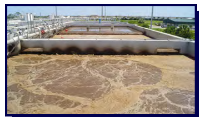
IFAS System - Aerobic AS Basin
