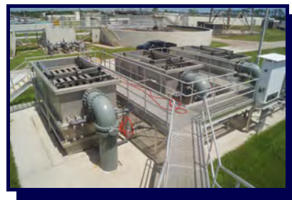
Tertiary (Disc) Filters - IFAS System
