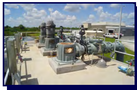
IFAS System - Transfer Pump Station
