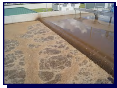
Aerobic IFAS Basin
