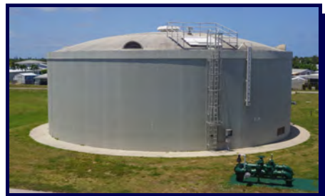
Reclaimed Water Ground Storage Tank
