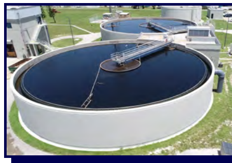
Secondary Clarifiers - Ox. Ditch System
