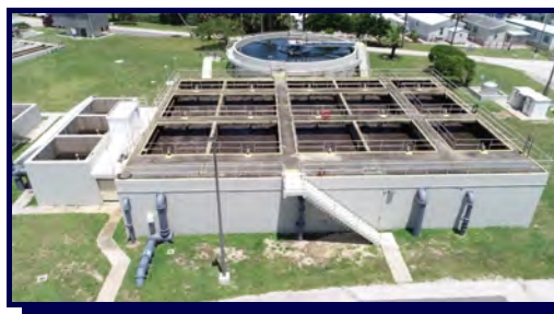
Conv. Activated Sludge Process System
