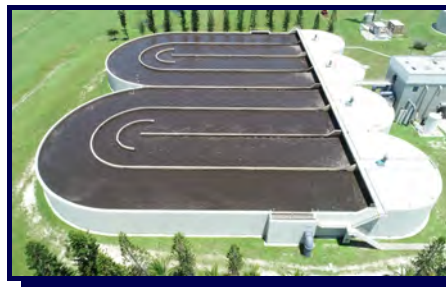
Carrousel Dual Oxidation Ditch System
