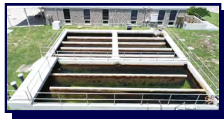
Chlorine Contact Chambers (CCCs)
