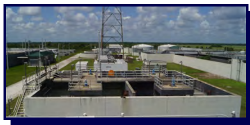
Carrousel BNR Treatment System: Anaerobic Basins
