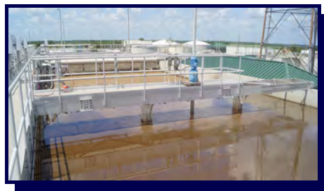
IFAS BNR System: Primary Anoxic Basins
