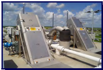
Mechanical Barscreens (3 mm)
