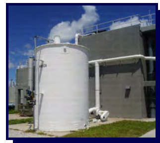
Pretreatment Structure Odor Control System
