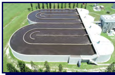
Carrousel Dual Oxidation Ditch System
