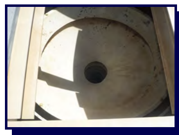
Grit Separator Unit (HeadCell)
