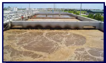
IFAS System - Aerobic AS Basin
