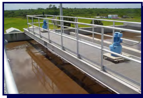
IFAS BNR System: Anaerobic Basins
