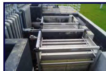
Tertiary (Disc) Filters
