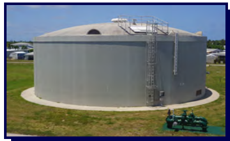
Reclaimed Water Ground Storage Tank
