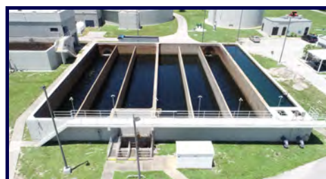
Secondary Effluent CCC/Equalization Tank
