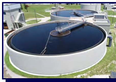
Secondary Clarifiers - Ox. Ditch System
