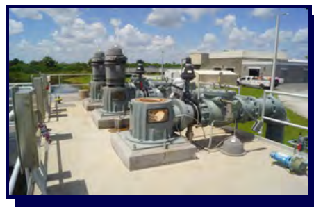
IFAS System - Transfer Pump Station
