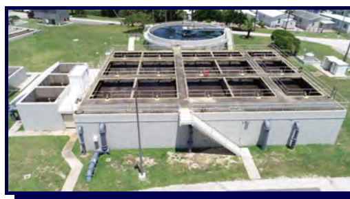
Conv. Activated Sludge Process System
