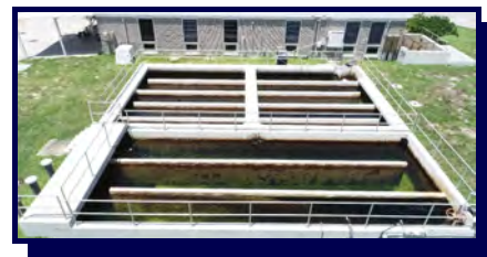
Chlorine Contact Chambers (CCCs)
