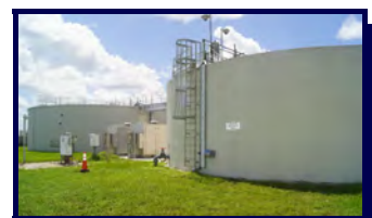
Sludge Holding Tanks
