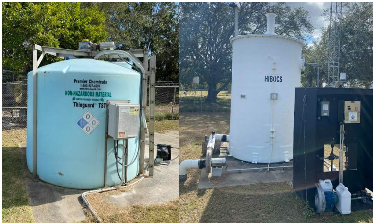
Figure 2-2 Thioguard Addition System (Left) and Biotrickling Filter (Right)
