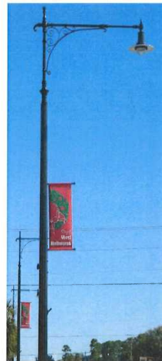
(Street lights installed in 2018 along US 192)
