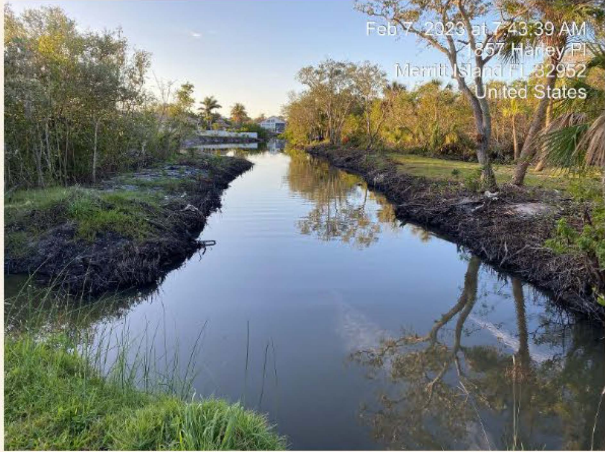
OLD CAUSEWAY RD LOOKING SOUTH AT OLD CAUSEWAY OUTFALL (ORANGE) NOTE: COUNTY'S MAINTENANCE ACTIVITY INCLUDED THE REMOVAL OF MULCHED VEGETATION AND ABOUT SIX (6) TO EIGHT (8) INCHES OF MUCK AT THE PIPE CROSSING, THEN TAPERING DOWN TO ABOUT 2 INCHES OF MUCK AT THE SOUTH PROJECT LIMITS. REMNANTS OF THE DEBRIS REMOVAL CAN BE SEEN ON THE LEFT (EAST) SIDE OF THE PHOTO FOR A SHORT DISTANCE DUE TO THE PROPERTY OWNER DREDGING ACTIVITY. TO THE RIGHT (WEST), THE PROPERTY OWNER INSTALLED SOD. TO THE SOUTHEAST, THE PROPERTY OWNER HIRED A CONTRACTOR TO DO SIGNIFICANT DREDGING AND EXCAVATION OF THE OUTFALL.
