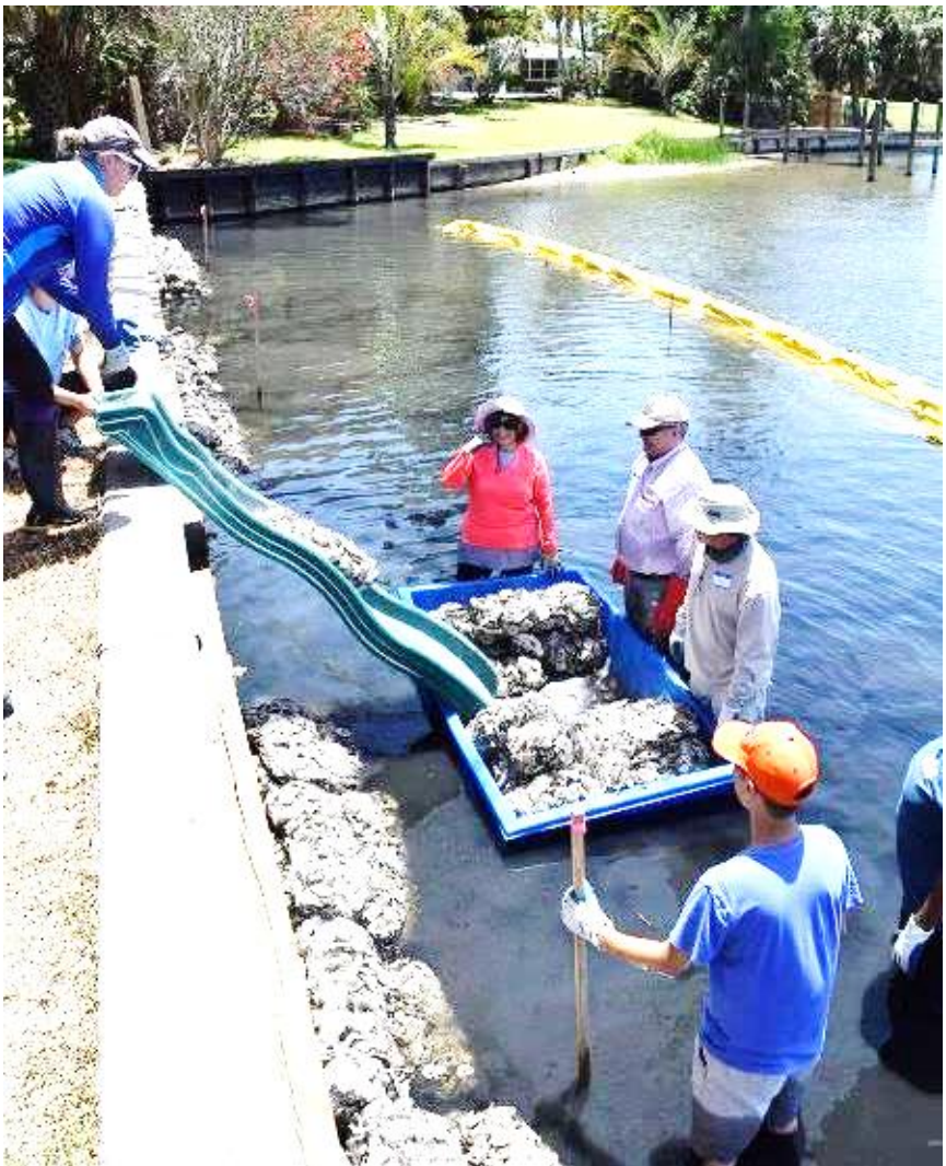
Brevard County Douglas Park Living Shoreline Demonstration site oyster seawall revetments and breakwaters
