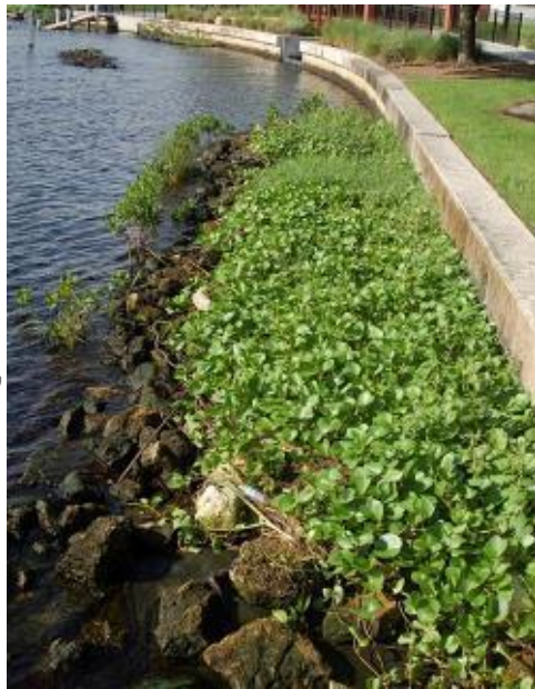
Redeemed seawall at FWC's Mosquito Lagoon Marine Enhancement Center Shoreline Demonstration Area New Smyrna Beach, FL (coquina planter, oyster bag planter, and rip-rap with native plants)
