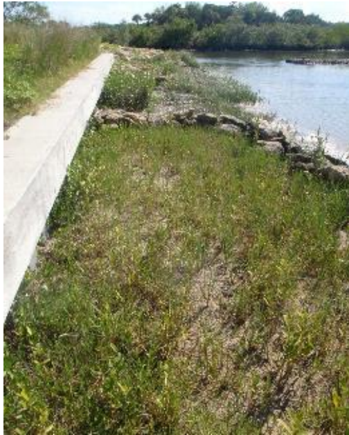
Redeemed seawall at FWC's Mosquito Lagoon Marine Enhancement Center Shoreline Demonstration Area New Smyrna Beach, FL (coquina planter, oyster bag planter, and rip-rap with native plants)
