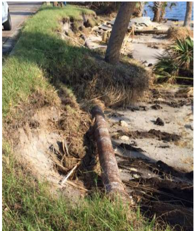
This image shows how erosion and flooding can begin to impair the integrity of roadways long before inundation occurs and also cause damage the underground utilities.
