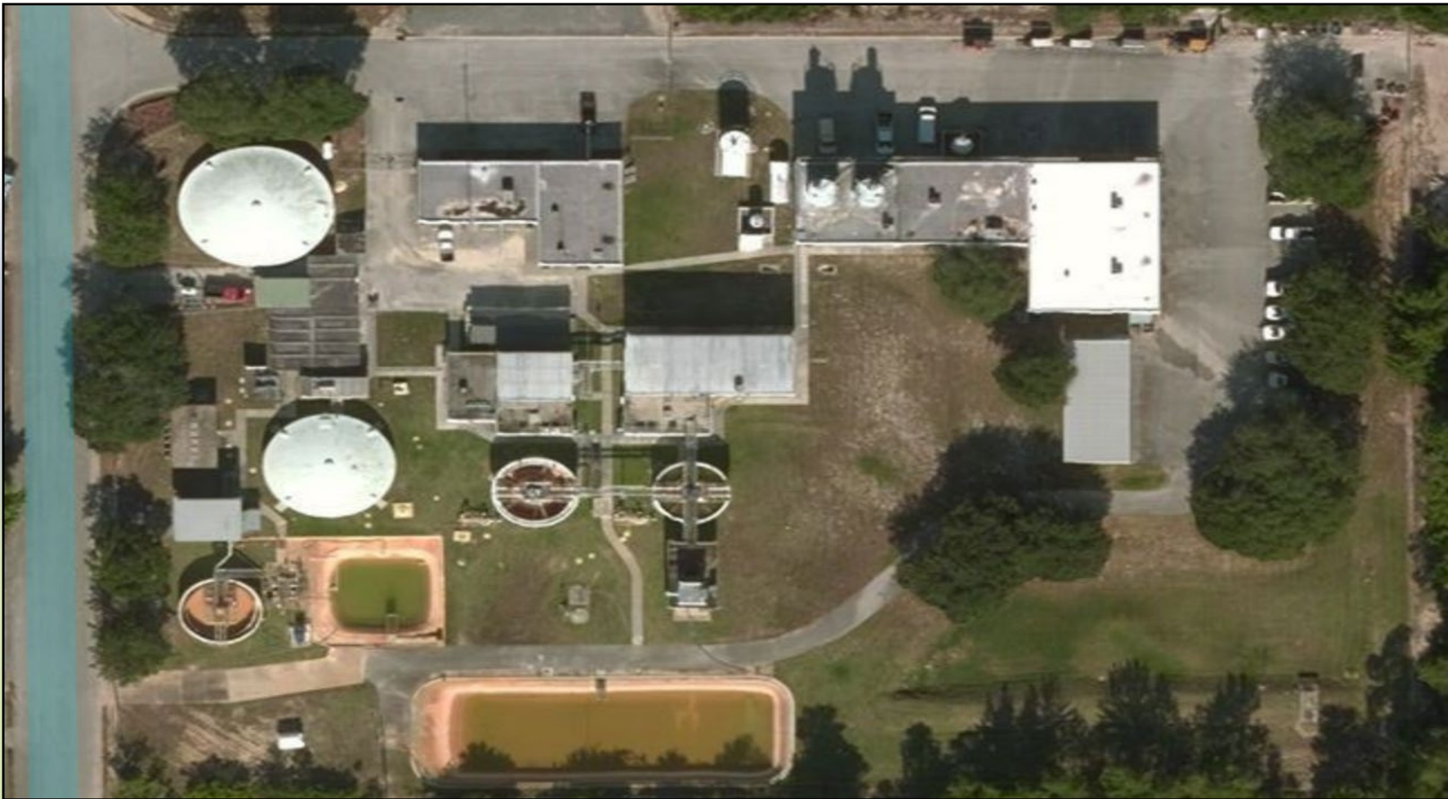
Figure 12 – Typical Water Treatment Plant
