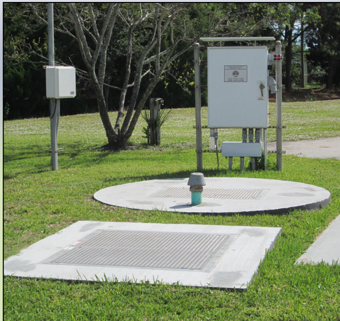
Figure 4 – Typical BCUSD Lift Station
