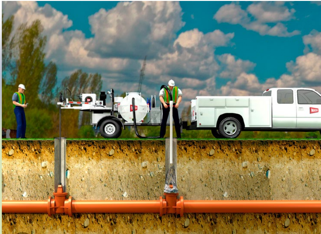
Figure 23 - Valve Exercising Example
