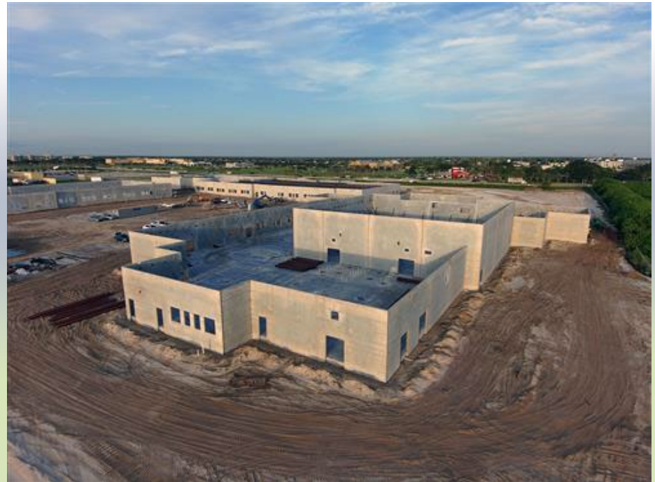
Figure 30 - Aerial View of Construction Mid County Middle School, Viera, FL
