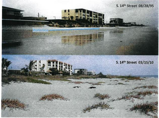
Photos above show south Cocoa Beach before and after the initial construction of the **North Reach Shore Projection** (beach nourishment) Project. Before the first nourishment of this project in 2001, the Cocoa Beach shoreline was seriously eroded and much of it had been armored with seawalls and rip-rap. After nourishment of the
