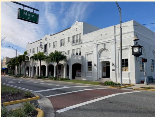
Launch Now Mixed Use Development almost complete
