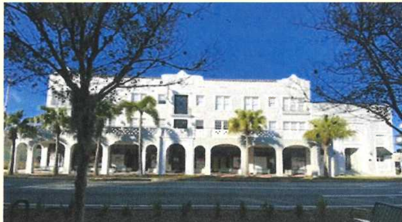
Launch Now Mixed-Use Development – almost complete
