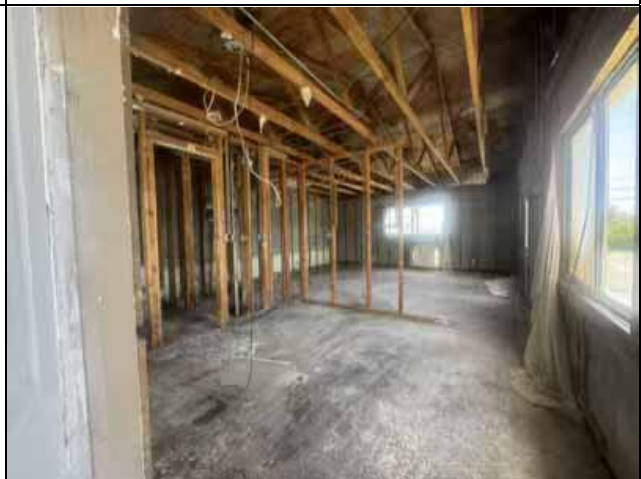
Interior of Second Floor Unit
