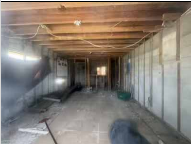
Interior of Motel/Old Barber Shop
