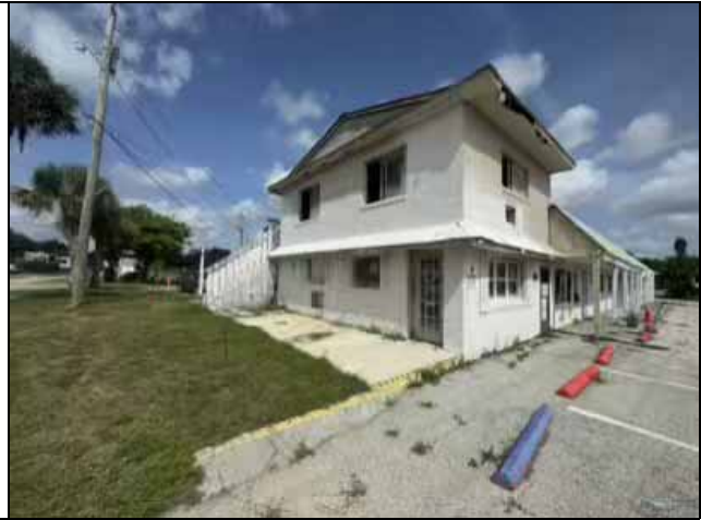
Front & Side – Southeast Corner
