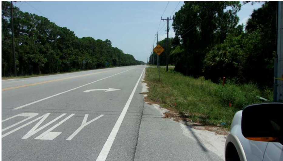
1. ADAMSON ROAD LOOKING SOUTH. SUBJECT FRONTAGE ON RIGHT
