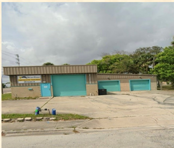
400 Garden Street – Vacant
