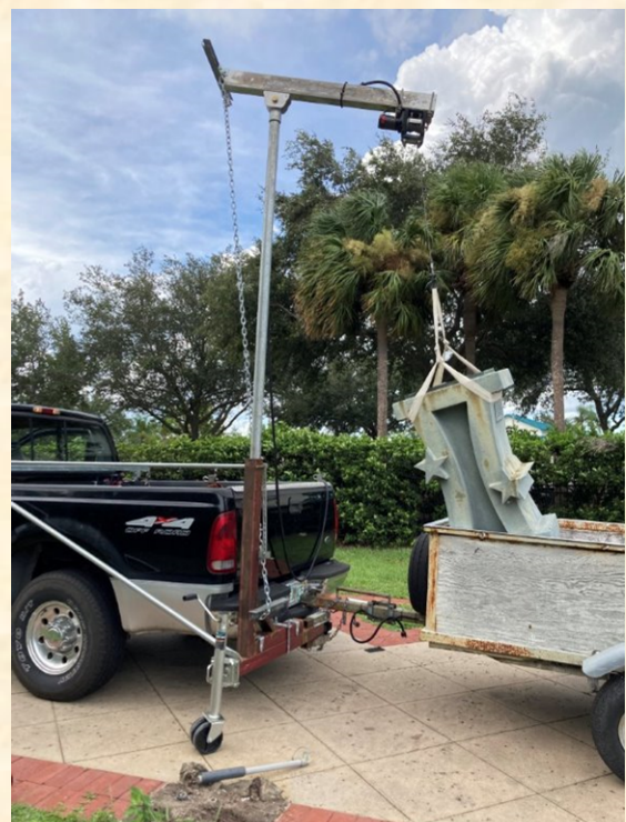
Removal for Restoration
