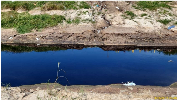
Leachate Mixing w/ Stormwater (E)
