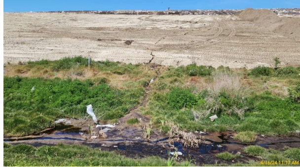
Leachate mixing w/ Stormwater (N)
