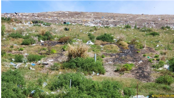
Waste Protruding South Side
