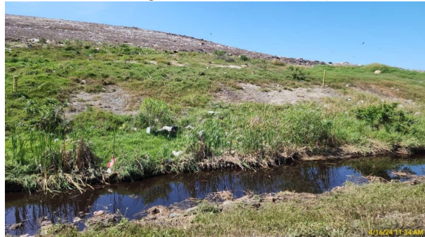
Leachate mixing w/ Stormwater (N)
