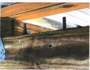
**(DS-18) Repair or Replace:** The main beam supporting the ridge beam and boat lift and motor was split in several areas. Recommend monitor and repair or replace as needed.
