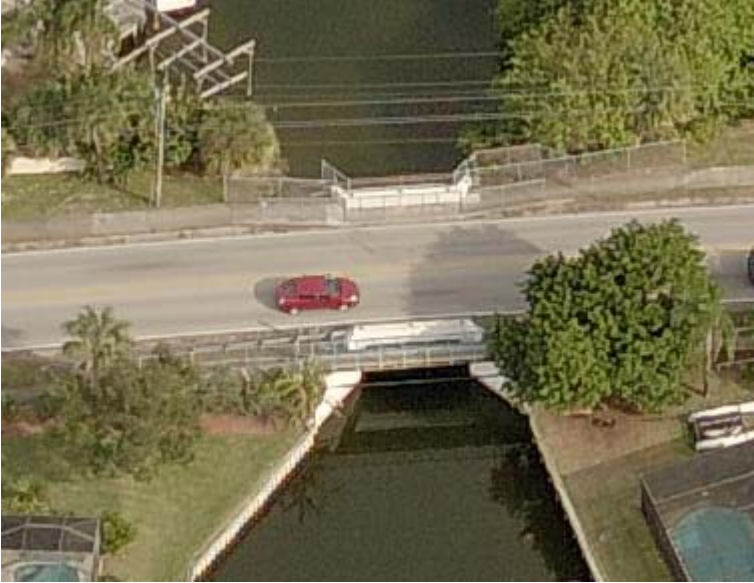
Constricted Roadway Segments over canals
