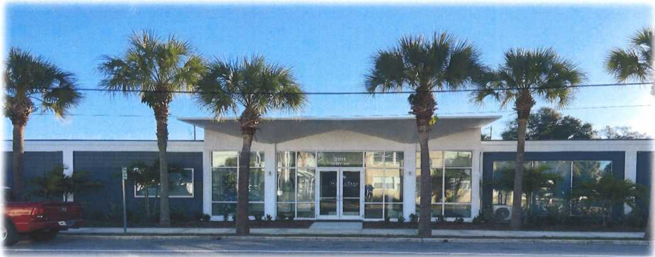
FIGURE 1 – 2101 WAVERLY PLACE FAÇADE BEFORE AND AFTER
