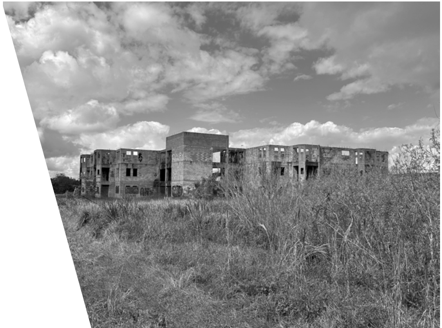
An abandoned, blighted multi-family housing project on North Courtenay Parkway, the area's most traveled north-south thoroughfare
