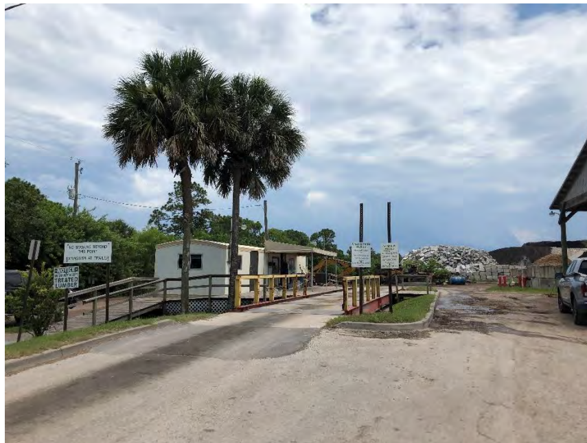
View of looking south at the manufactured building serving as the onsite office and adjoining weight station.
