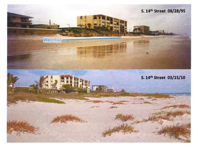
Photos above show south Cocoa Beach before and after the initial construction of the North Reach Shore Projection (beach nourishment) Project. Before the first nourishment of this project in 2001, the Cocoa Beach shoreline was seriously eroded and much of it had been armored with seawalls and riprap. After nourishment of the North Reach, waves could no longer reach the seawalls, and this allowed dunes to develop with wind-blown sand, provided by the project, collecting around native plants.
